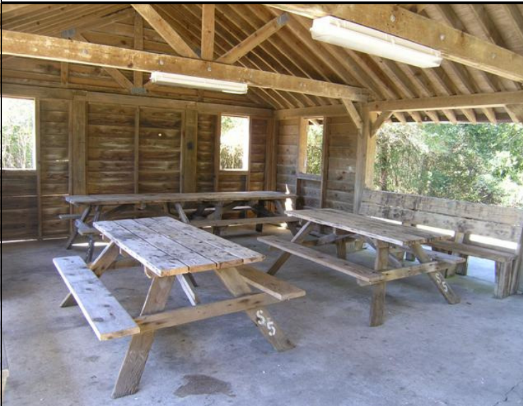
Inside Shelter B5 (Photo shows half of shelter)
