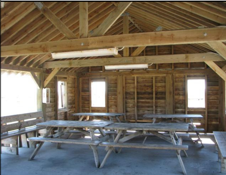
Inside Shelter B3 (Photo shows half of shelter)
