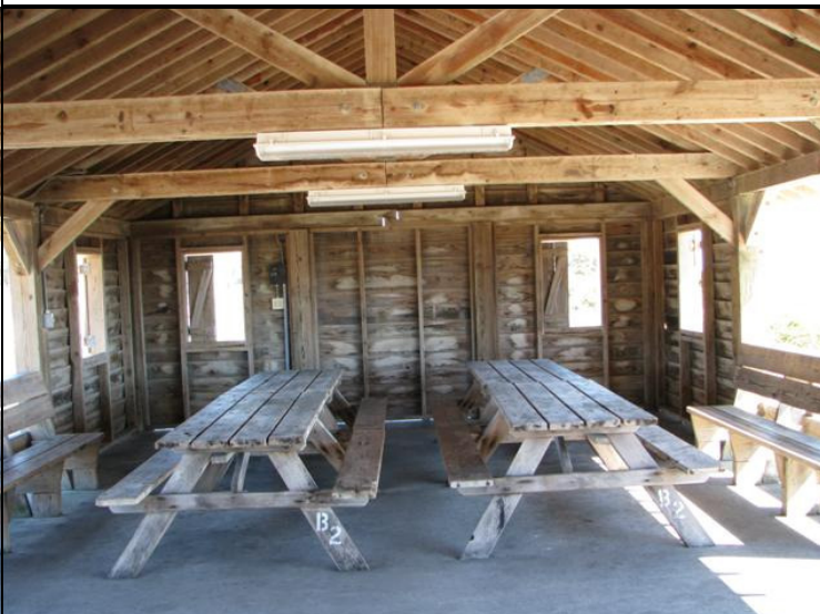
Inside Shelter B2 Photo Shows Half of Shelter
