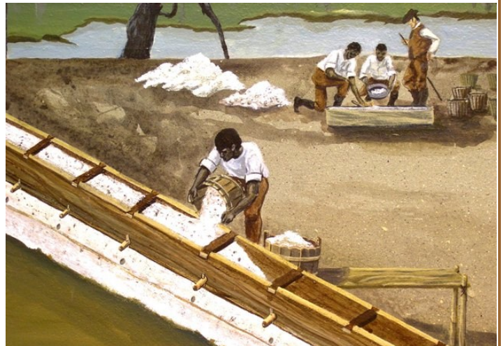
A tabby wall under construction, showing the design of the wooden form used to create each layer.
