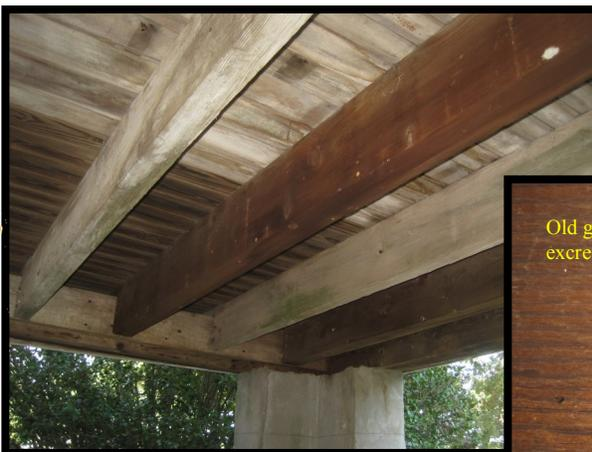
Carpenter bees attack dry, exposed wood and can often be seen hovering under the eaves of houses or the undersides of porches such as the underside of the historic porch of Redcliffe Plantation's mansion (left).
