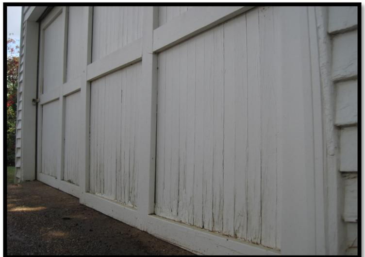
Water damage to the lower portions of the 1935 garage doors.
