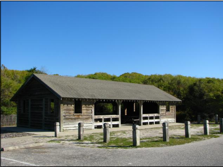
Shelter B6 Front View
