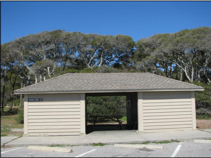
Shelter 2 Front View
