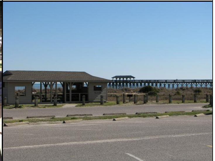
View from Front of Shelter 2
