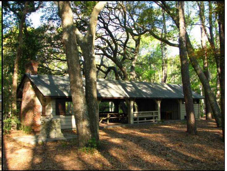
View from Back of Shelter 1
