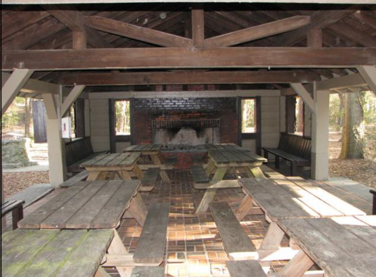
Inside Shelter 1 Photo Shows Little over Half of Shelter
